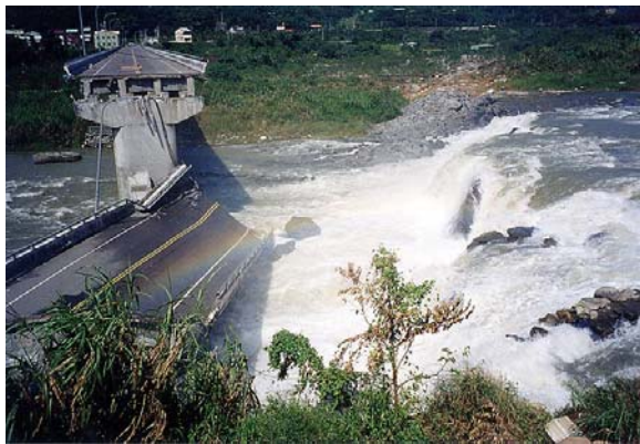
Figure 2.17. Bei-Fong bridge and fault-created Waterfall
