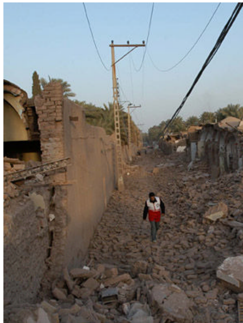
Fig. 6.2: Poles remaining upright in debris (2003 Bam Earthquake, Iran)
