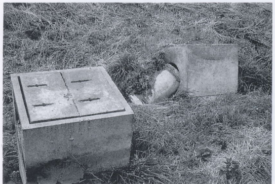
写真 4.4.33 今金町豊田の農道の被害(12) 浮き上がった農業用配水枡 Water distribution device lifted up due to liquefaction (12)
