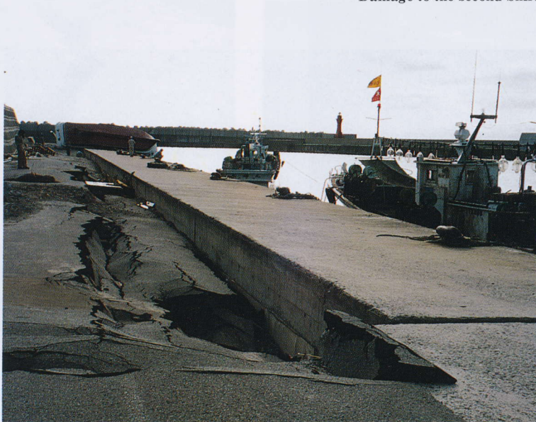
写真 4.2.18 須築漁港の船着場の被害状況 Sutsuki fishing port damaged by tsunami and severe tremor
