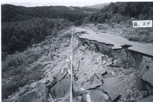
写真 4.5.1 北檜山北の町道盛土の被害 (1) Damage to road embankment (1) (Kitahiyama town)
