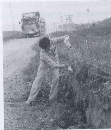
写真 4.3.9 堤防の河心側への滑動と沈下(兜野橋近傍) Settlement of left embankment associated with its lateralspread (near the Kabutono bridge)
