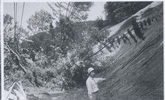
写真 4.1.4 流れ盤型の斜面崩壊 ([24] 地点) Rock-slide on layer boundary (Point [24])
