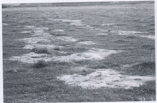
写真 4.3.10 堤内地にみられる液状化のあと Line of sand cones on river reservation near the left embankment (Shiribeshitoshibetsu river)
